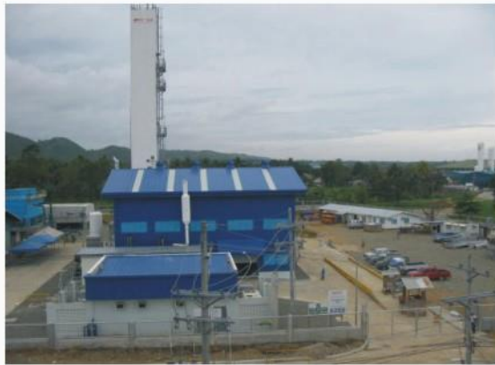
Air Separation Unit Plant (ASU) Southern Industrial Gases, Inc. (now Linde Southern Phils., Inc.) CIPDI, Buanoy, Balamban, Cebu Land Development, Architectural, Plumbing, Civil & Structural Works Building & Occupancy Permits Acquisition
