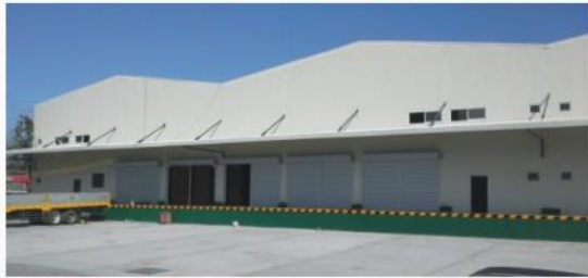
Greencross Warehouse Dasmariñas, Cavite Masonry & Painting Works
