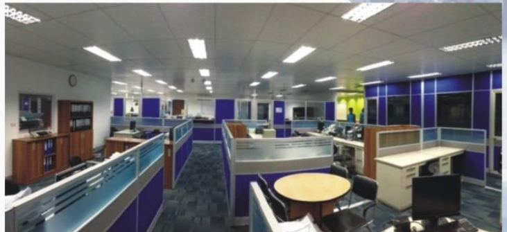
Headquarters Office Renovation NEP Logistics, Inc. Laguna Technopark Inc. Binan, Laguna Electrical & Architectural Works / Fit-Out
